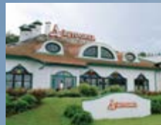
ARNWIESEN SERVICE AREA, A2 MOTORWAY, GLEISDORF (AUSTRIA)
