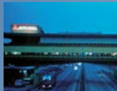
AUTOGRILL® BRIDGE CANTAGALLO, A1 MOTORWAY, BOLOGNA (ITALY)
